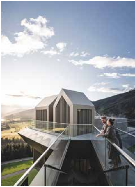
ICONIC ARCHITECTURE: The 'Heaven & Hell' Sky spa is an astounding feat of architecture
